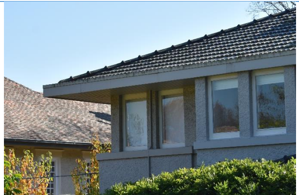
Detail of upper floor fenestration and overhanging boxed eaves (source: Extent Heritage Pty Ltd, 2021).
