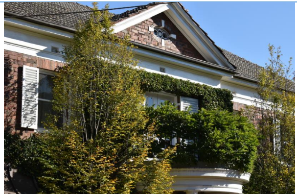
Detail of gable end with oval shaped bullseye window (source: Extent Heritage Pty Ltd, 2021).
