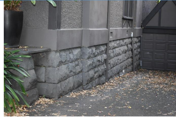
Bluestone foundation, eastern elevation (source: Extent Heritage Pty Ltd, 2021).
