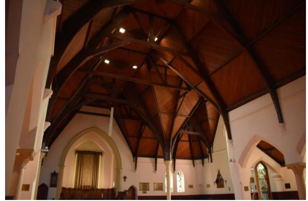
Overview of timber vaulted ceiling and trusses (source: Extent Heritage Pty Ltd, 2022).
