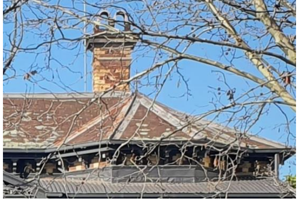
Detail of the chimney and double fronted hipped roof form (source: City of Stonnington, 2020).
