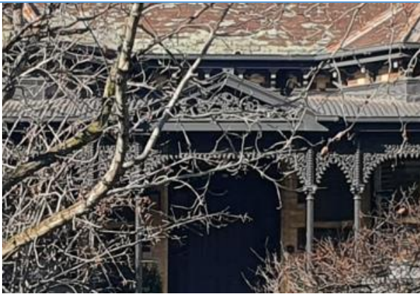
Detail of triangular verandah pediment (source: City of Stonnington, 2020).
