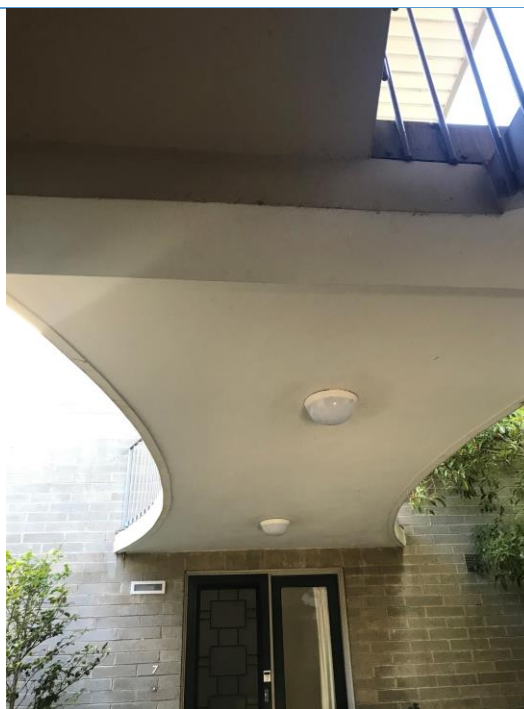
Underside of concrete and steel connecting walkway (source: Extent Heritage Pty Ltd, 2021).
