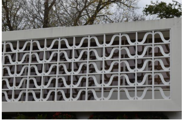
Detail of steel screen (source: Extent Heritage Pty Ltd, 2021).
