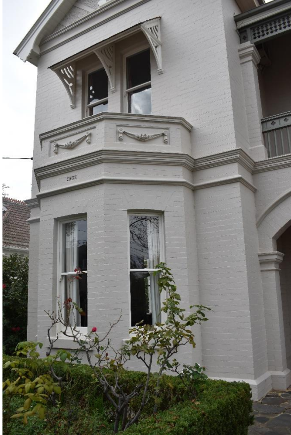
Detail view of projecting bay window below the front gable (source: Extent Heritage Pty Ltd, 2021).
