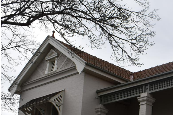
Detail view of front facing gable roof form and terracotta tiling (source: Extent Heritage Pty Ltd, 2021).
