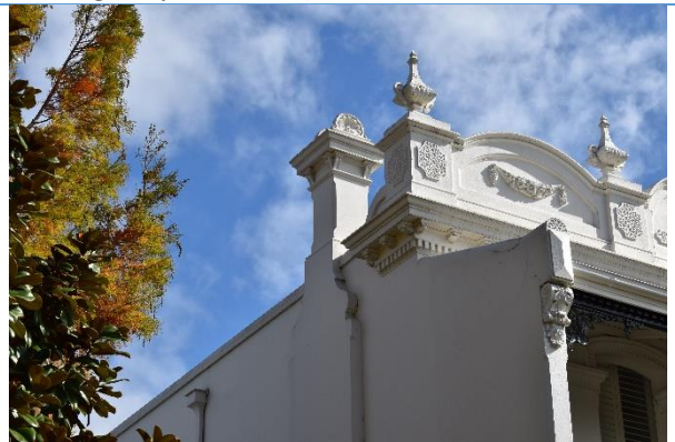
Detail view of south-east parapet corner and profiled chimney (source: Extent Heritage Pty Ltd, 2021).
