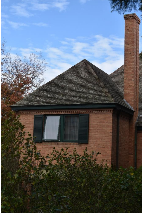
Detail view of the upper level double awning windows with timber louvred shutters (source: Extent Heritage Pty Ltd, 2021).
